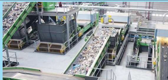
Figure 1: Conveyors transporting C&D waste material
