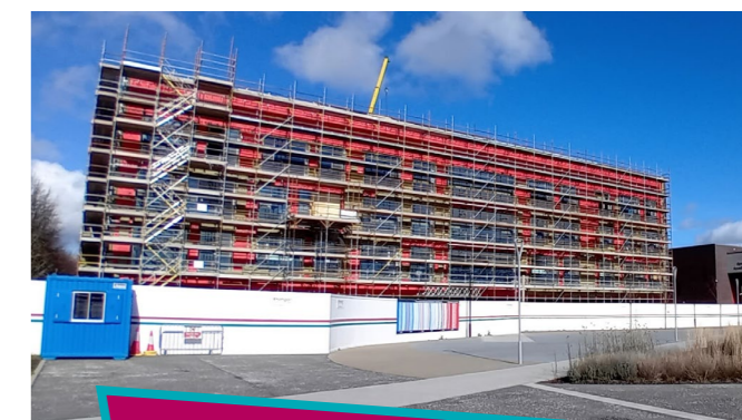
HEPPP North Building on Tallaght Campus under construction
