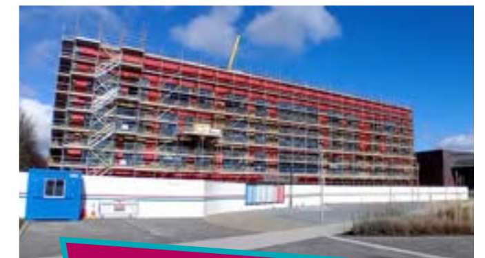
HEPPP North Building on Tallaght Campus under construction
